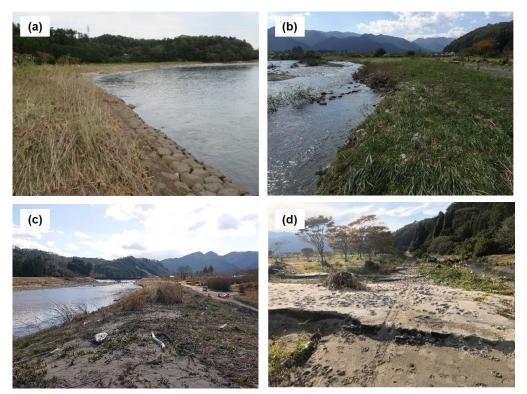
Figure 6. Photos showing the situations of riverside areas (a) River revetment exposed due to river bank erosion caused by the passage of Typhoon No. 19, (b) The same river revetment before being eroded (a photo taken from the opposite side on September 28, 2015), (c) Sediments deposited along the Niida River, (d) Sediment deposited along the branch river north of the park
